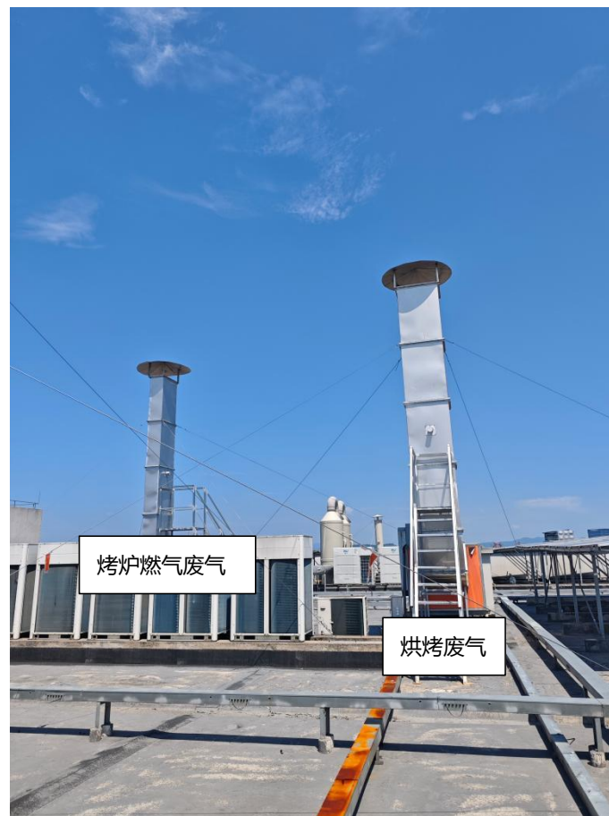
燃气废气排气筒 DA002、DA003；烘烤废气排气筒 DA004、DA005
